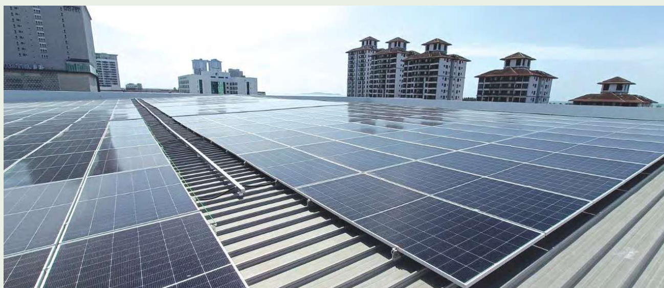
► Solar panel installation at Mahkota Parade
